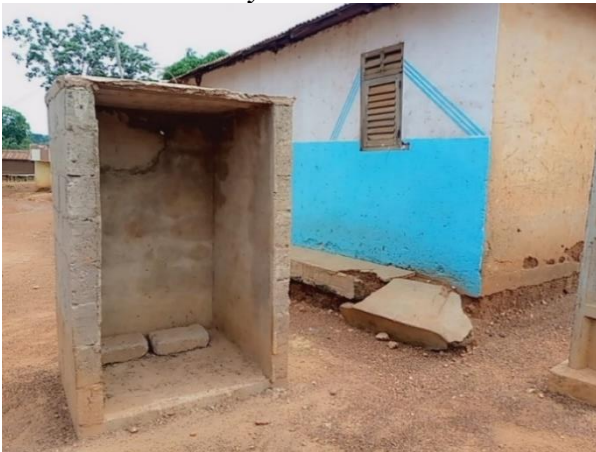
Picture 1: An electricity niche at N’Zuassé
