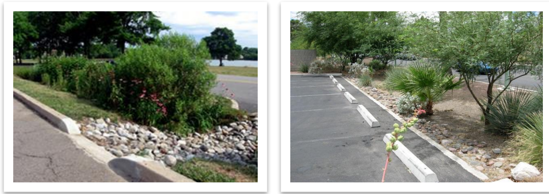
FIGURE 2: PAVEMENT RAINWATER HARVESTING [6] [7]
