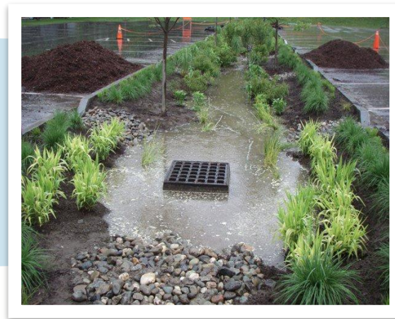
FIGURE 4: RAINWATER GROUND CATCHMENT [9]
